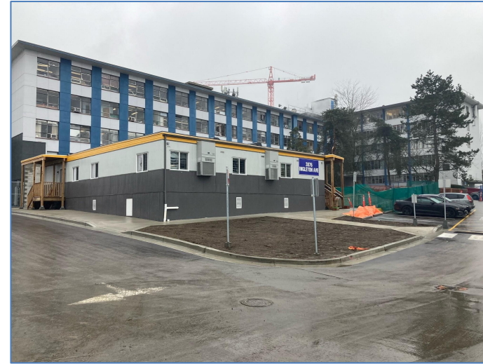
Temporary Administration modular
