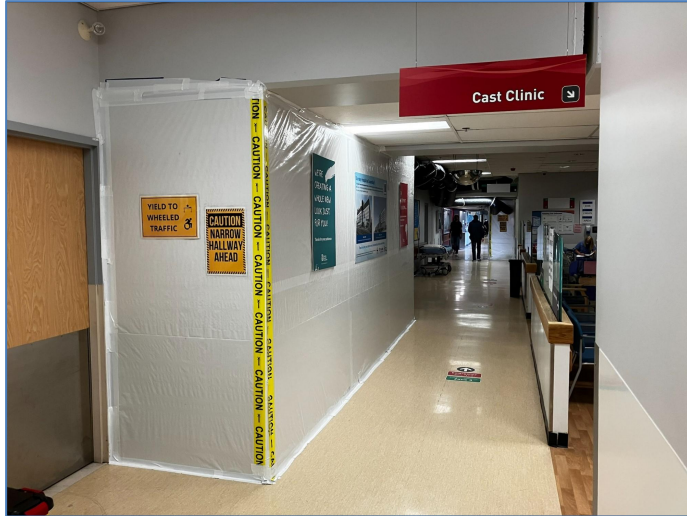
Construction hoarding near Emergency Department
